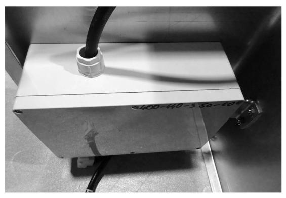
The box can be serviced by removing the screws on the outside with only the foot removed.
